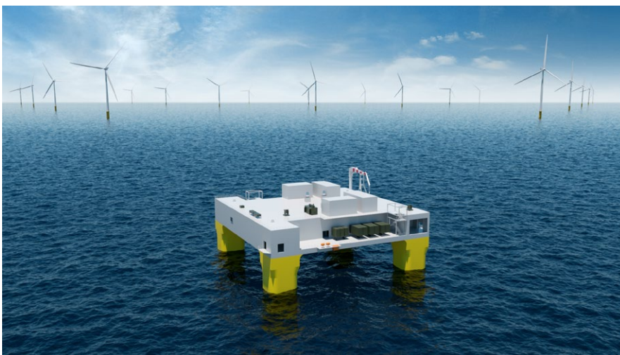
Figure 4: Floating HVAC station. Left: A general concept from Aibel for 500–1500 MW. Right: The first realized floating substation in the Fukushima floating wind test park in Japan.
