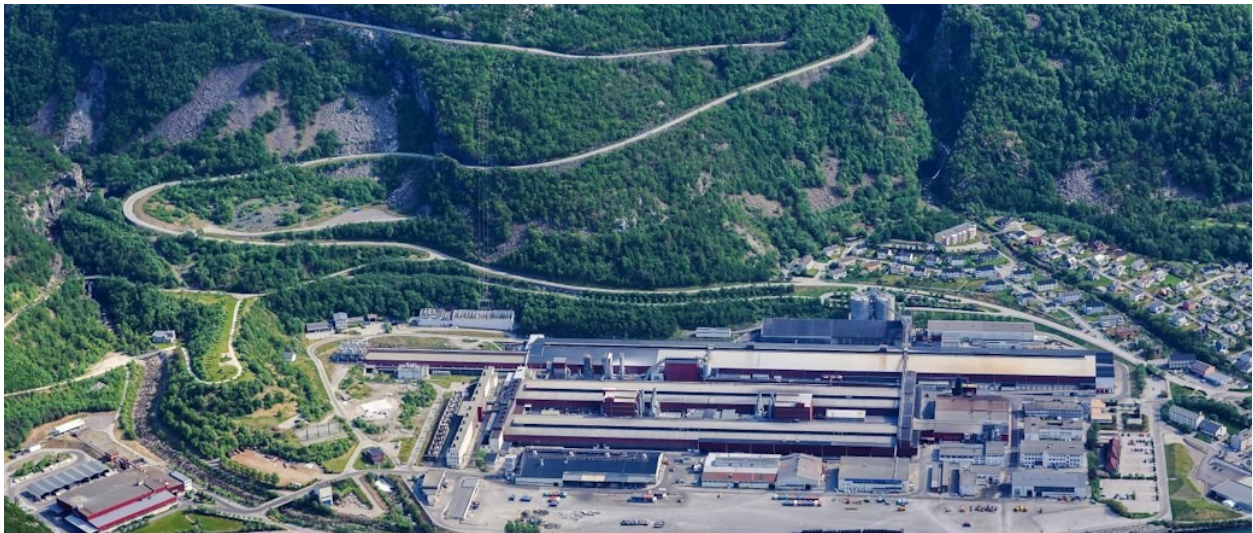
Figure 7-3: Air view of the Hydro Aluminium plant (metallverk) in Øvre Årdal.
